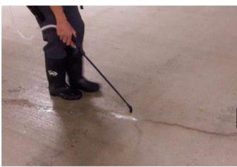
• If there are specific cracks that are leaking, flood cracks with a 15% solution of CMA Accelerator
