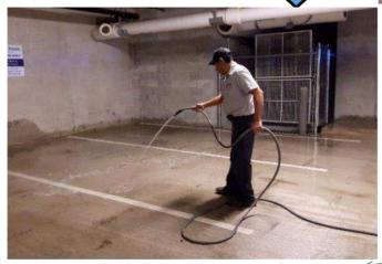
• Apply a generous amount of water to the entire surface. Have someone watch below for any excessive amounts of water leaking through the floor. Use about the same amount of water as product applied.
